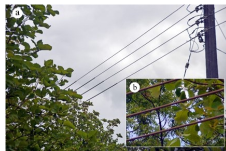
Fig. 2. Short segments of uninsulated electric cables that coursed near tree branches (a) were encapsulated in PVC water pipes (b) as a supplementary means to prevent monkeys and other arboreal mammals from suffering electrocution at sites where the trimming of tree branches was irregular.
