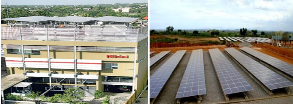
Figure 1. A solar roof (25 kW) on a commercial building in Colombo and one of the two solar farms (500 kW each) installed in Sri Lanka for initial training and promotional purposes.
